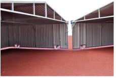
The garage elements are screwed together with metric screws only, without riveting or welding.
