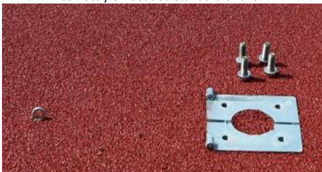
Correctly embedded standard anchor
