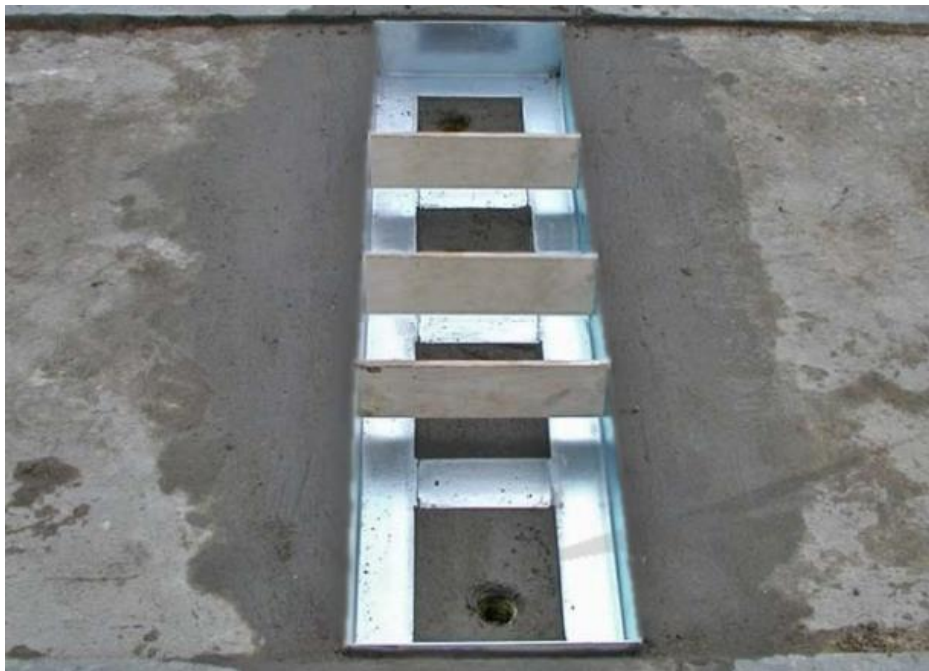
Image no. 1. Installed tray secured with spacing boards
